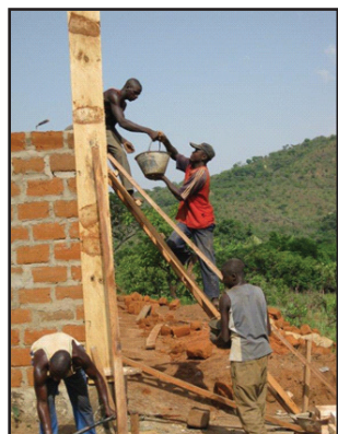
Pouring the corner posts, one bucket of cement at a time
